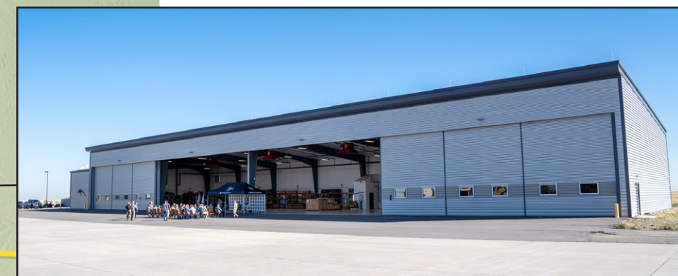
This new 21,600-square-foot unheated aircraft storage hangar was officially opened on Oct. 3, 2024, for the Army Aviation Support Facility.
